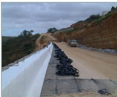
Figure 8 - Paralink in combination with Terramesh System
