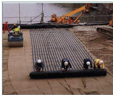
Figure 10- Paralink in combination with Terramesh System
