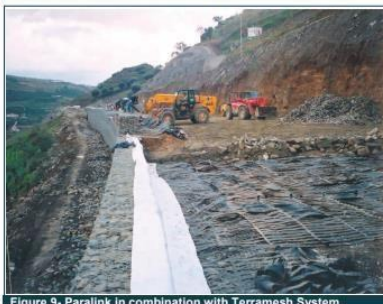
Figure 9- Paralink in combination with Terramesh System
